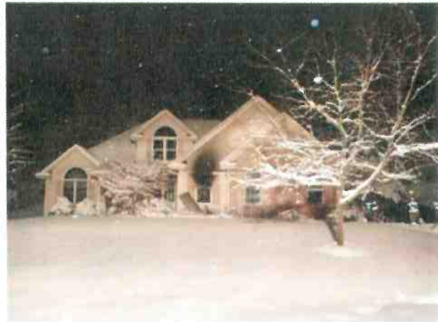
Right: Residential garage fire during a snow storm. A quick response and fire attack extinguished the fire quickly.
